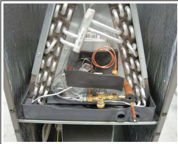
FIGURE 16. Coil Installed on Support Brackets
