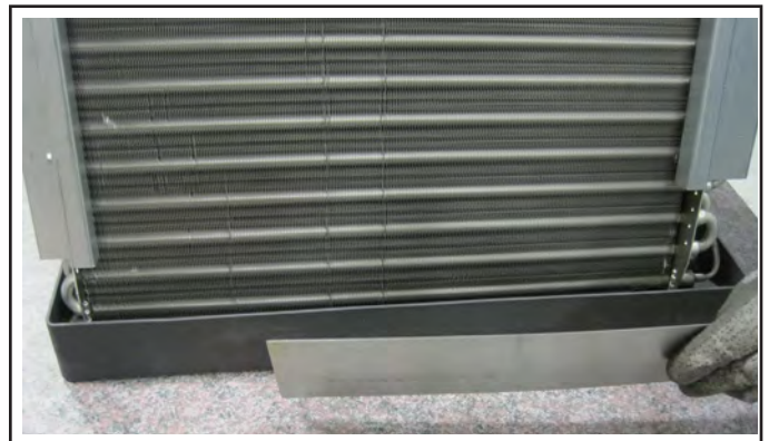
FIGURE 10. Slab Shield Positioned for Installation
